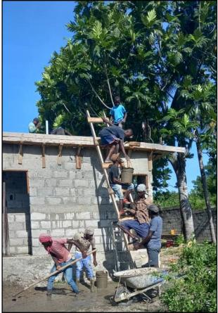
The community came together to pour a concrete roof over the bathroom. As you can see, much of the work is done by hand. Men worked hard as a team to complete the difficult task
